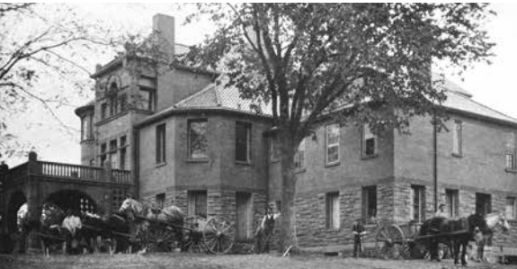
The Coykendall Mansion, designed by Calvert Vaux, under construction on West Chestnut Street c. 1895.
